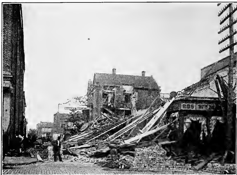
FIG. 287. — Destruction of buildings during the Charleston earthquake in 1886. (Hillers, U. S. Geol. Survey.)
